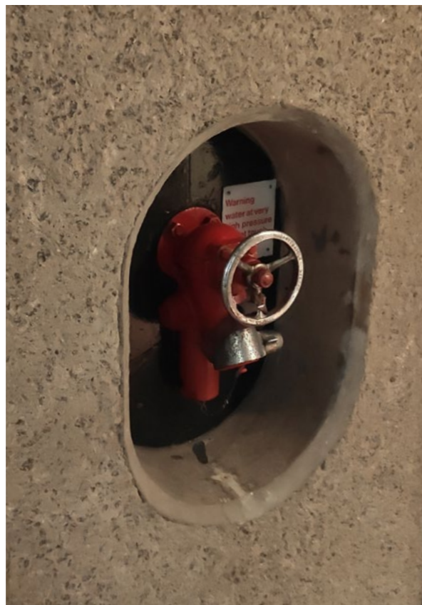
Recessed wet riser in concrete wall
